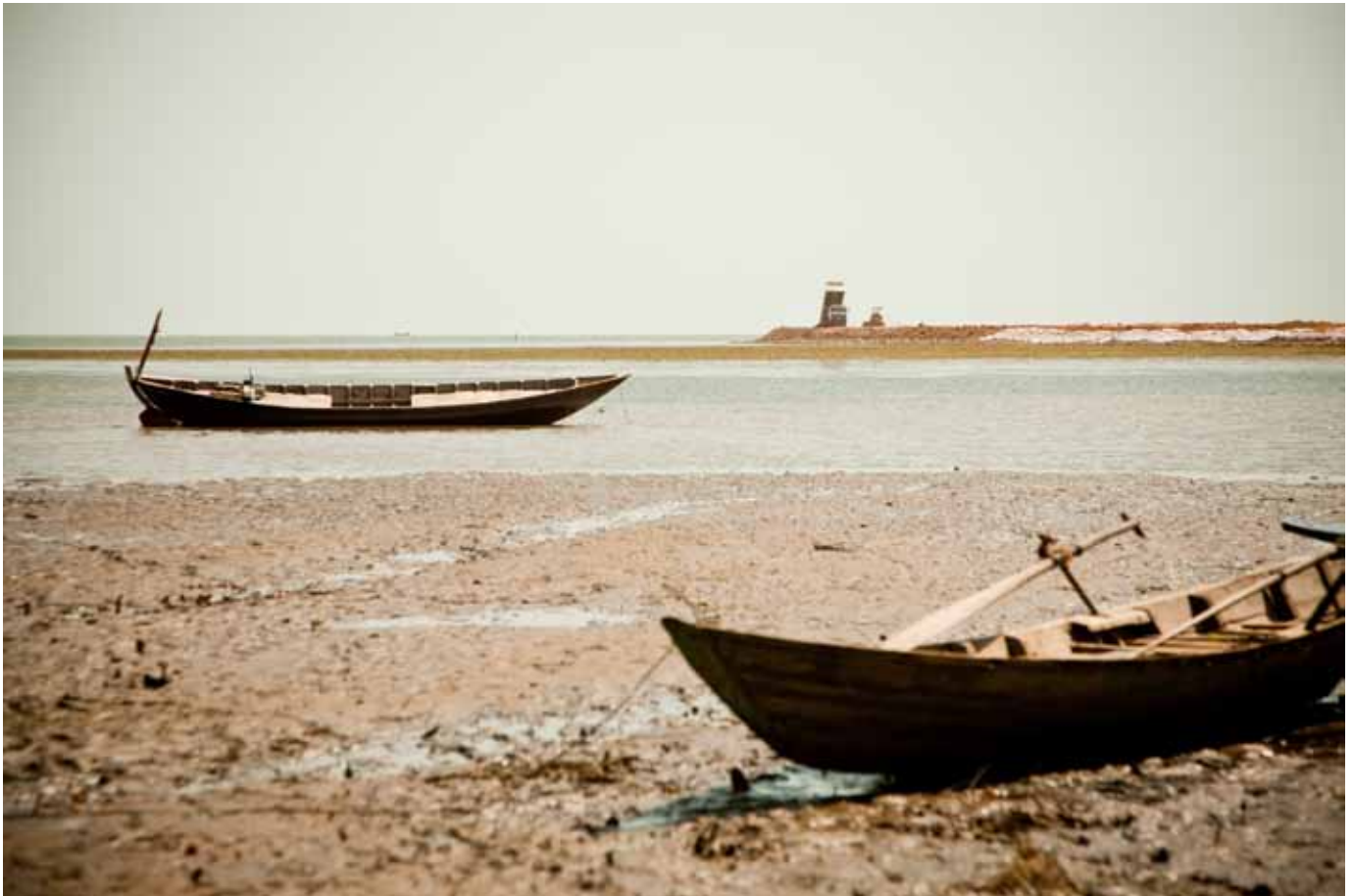
Trucks from the Wing Huor Co. fill in coastal waters of Kampot to construct Cambodia's second deep water port and a special economic zone where investors receive impressive tax-free status. Photo by Peter Schrock
