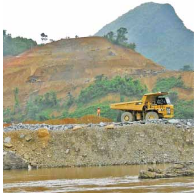
Construction of the Xayaburi Dam in Laos has begun.
