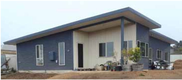
Manna Gum's new home (cont.): passive solar design is a simple concept that combines using a northward orientation, internal thermal mass, eaves, double glazing and heavy insulation to provide warmth in winter and coolness in summer; (above) view from the street - the house opens to the north to capture the winter sun; (right) living space - heats by sunlight when the sun is out and wood heater when it is not.
